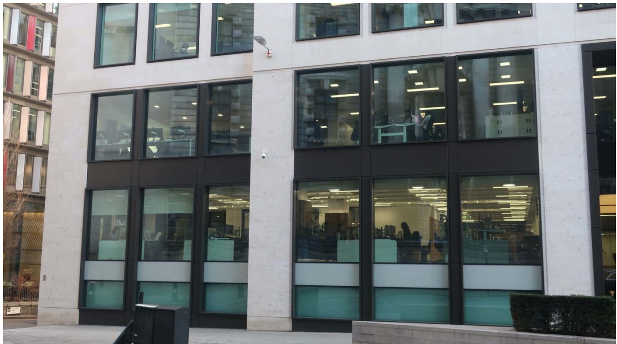
Photograph 2 – Front elevation showing the 2017 installed infill curtain walling.
