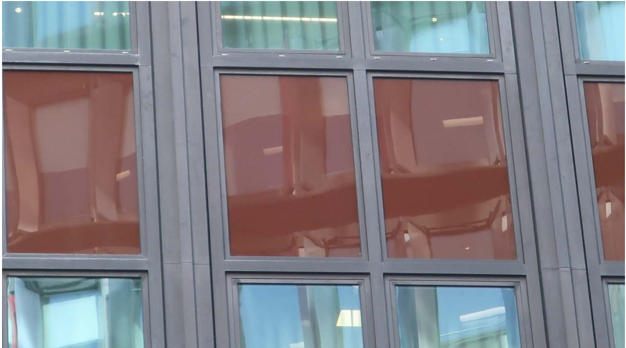
Photograph 9 – Original curtain walling spandrel panel at floor level.
