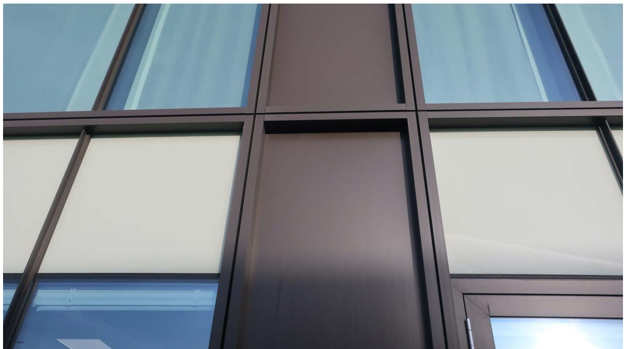
Photograph 16 – Close view of the 2017 installed curtain wall at Level 8 & 9.
