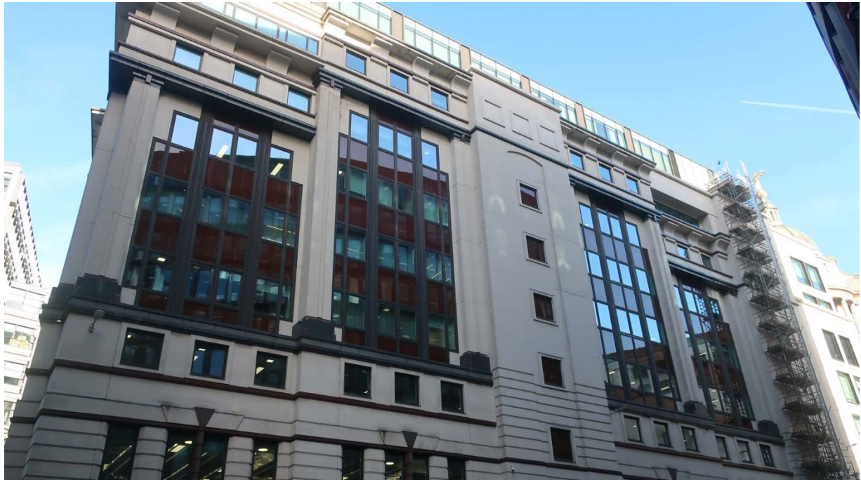
Photograph 7 – General view of the south elevation.
