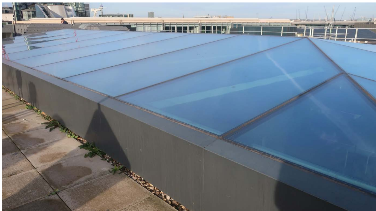
Photograph 17 – General view of the glazed atrium roof.
