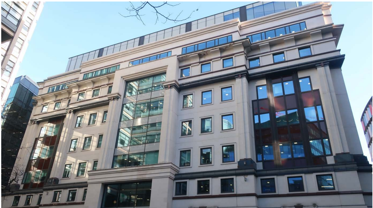
Photograph 10 – General view of the rear west elevation which is mostly original other than new stonework, windows and curtain walling at high level.
