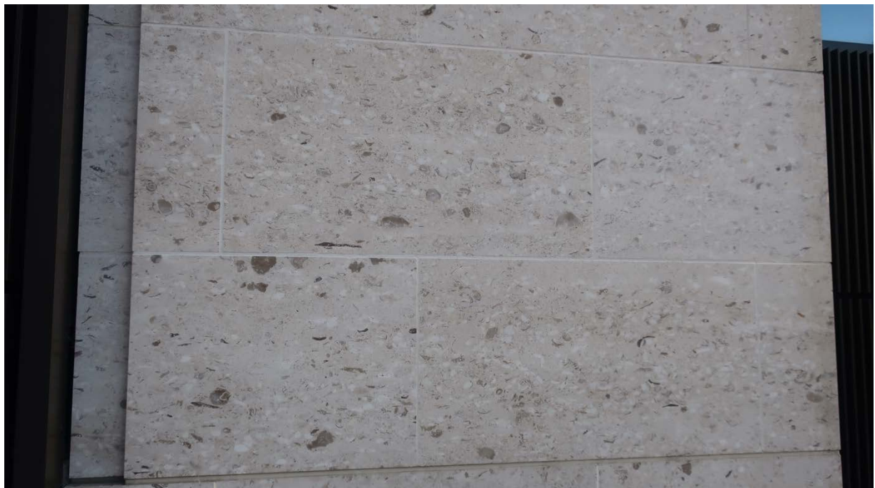
Photograph 4 – Close view of the 2017 installed Moleanos stonework in a satisfactory condition.
