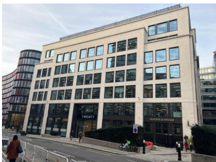
Photo of the front elevation.
