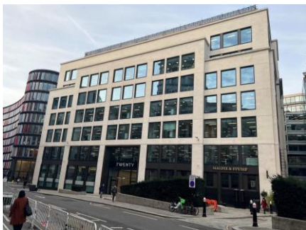
Photo of the front elevation, east facing
