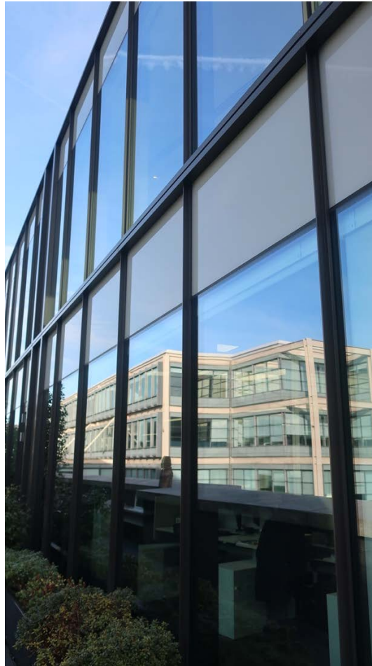
Photograph 15 – 2017 installed curtain wall at Level 8 & 9.
