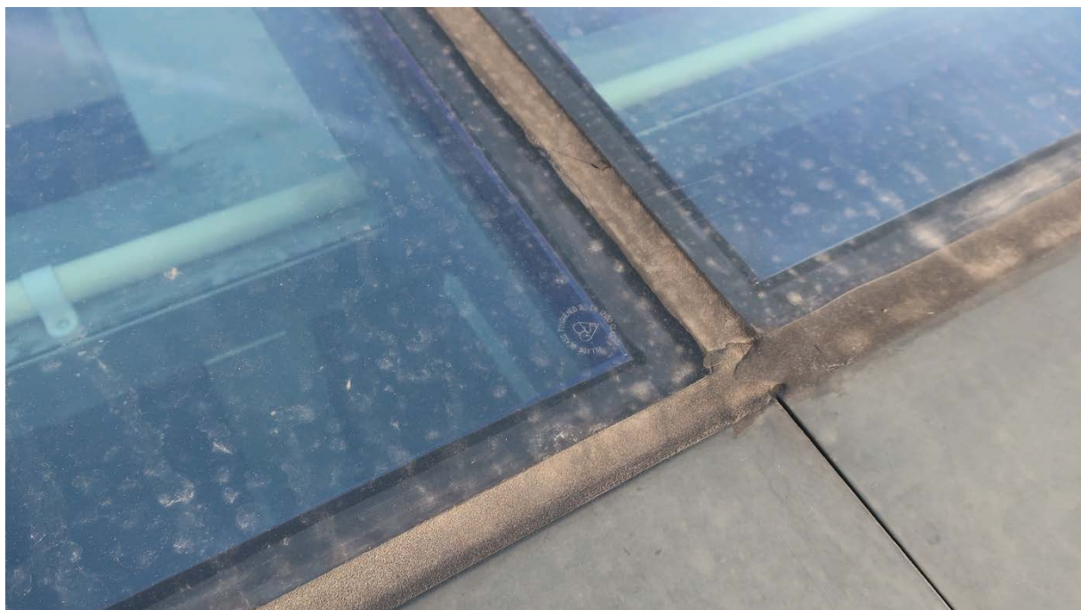
Photograph 18 – Close of the atrium roof silicone seals in a satisfactory condition.
