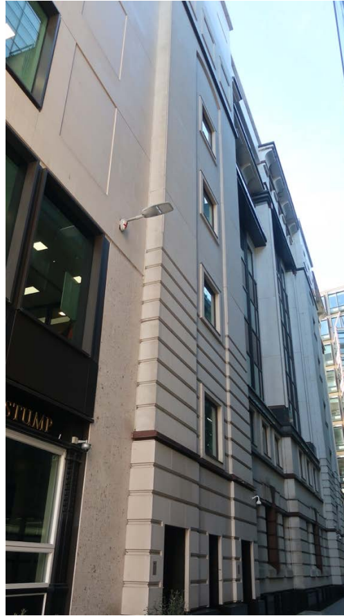
Photograph 5 – North elevation. (2017 stonework on the left and original stonework on the right)
