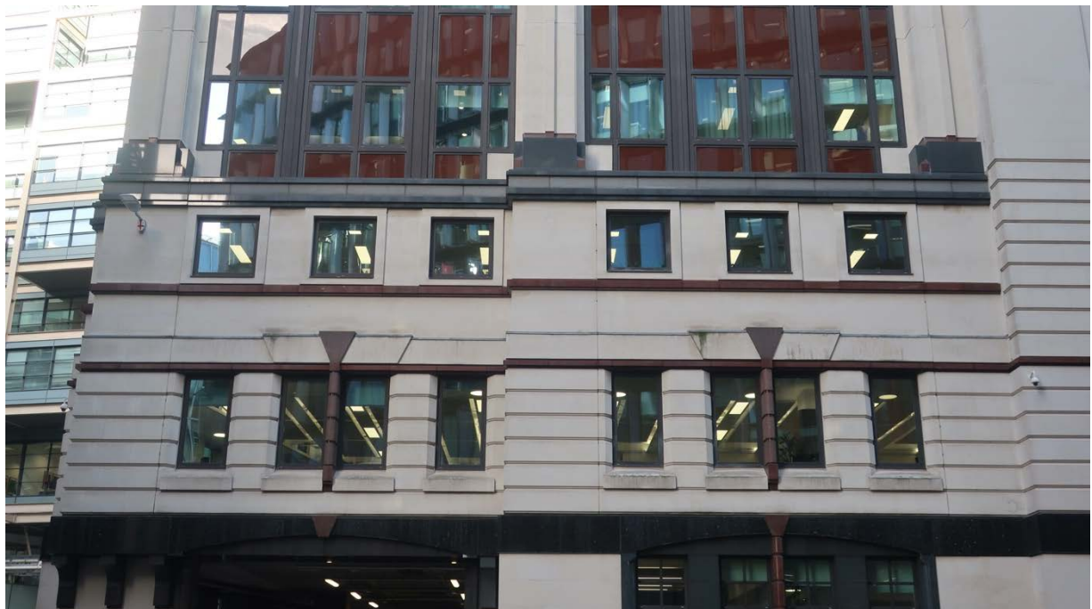
Photograph 8 – Part view of the south elevation showing the original stonework and windows.
