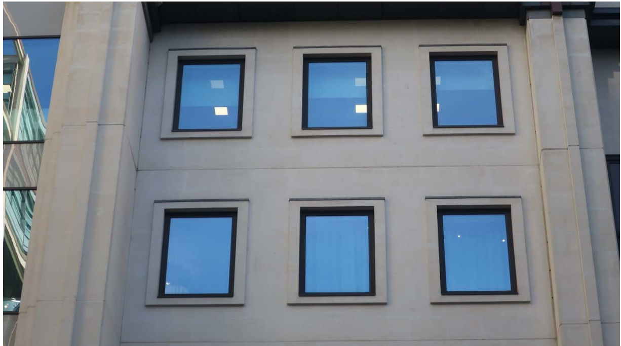
Photograph 13 – Rear west elevation showing the original stonework and windows.
